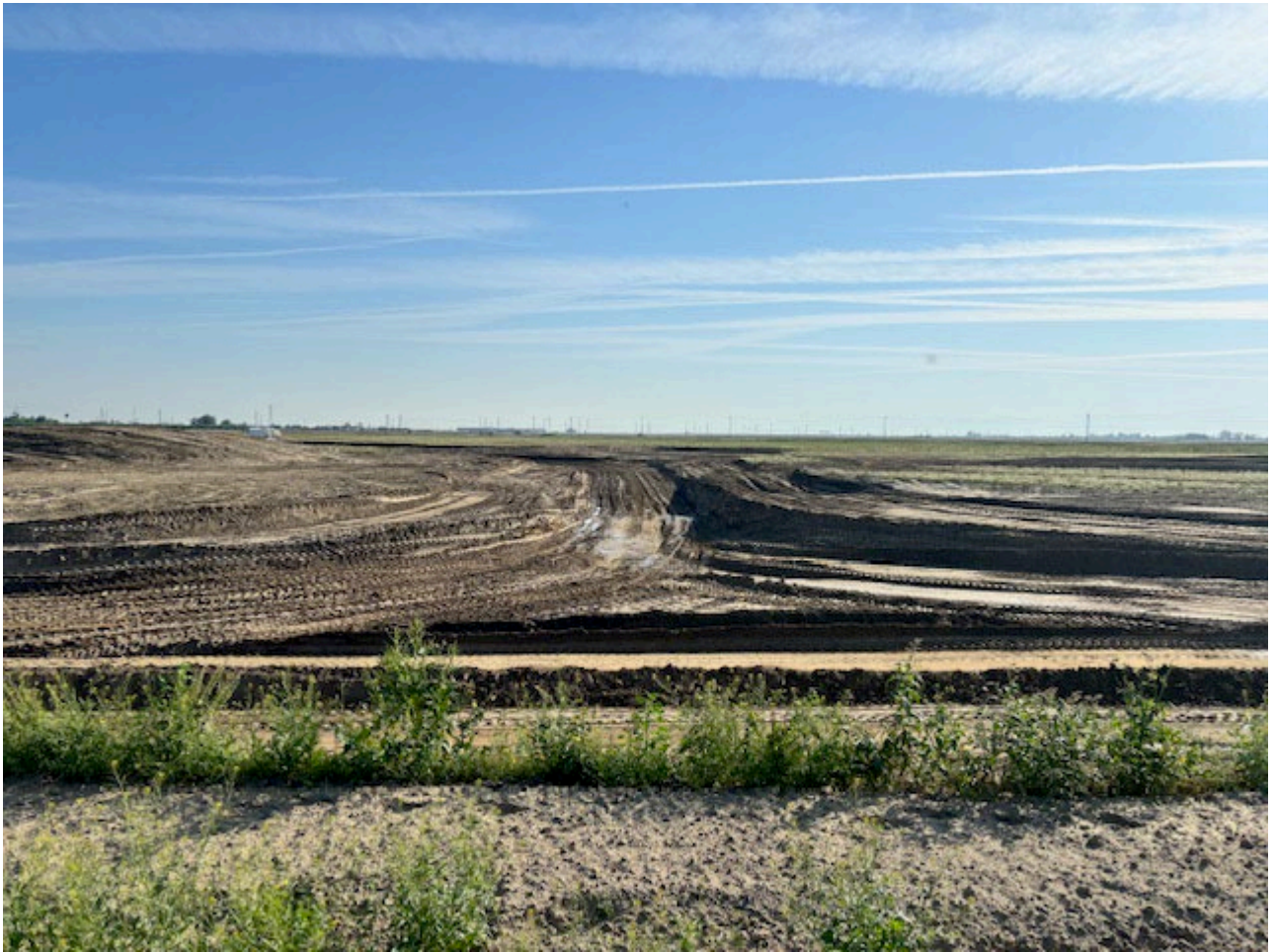
Excavation of Keyway for Levee between Basins 1 and 2
