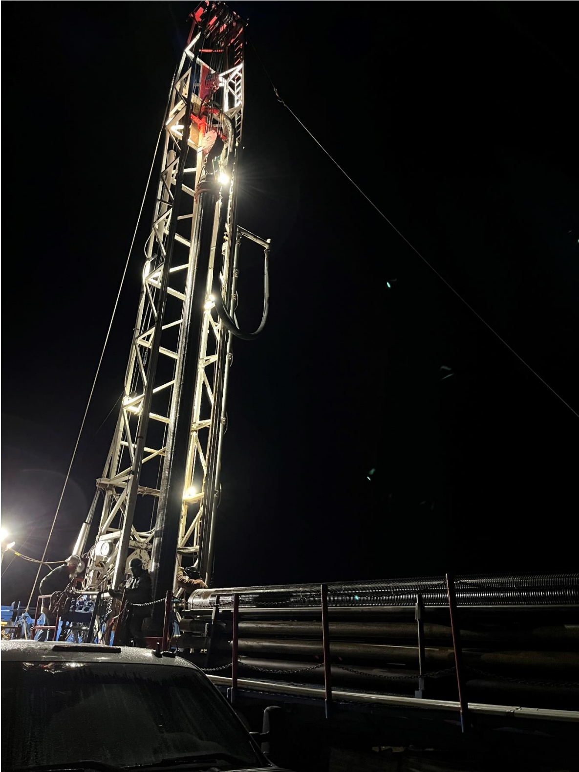
Figure 2: Construction of McCaslin 1 well
