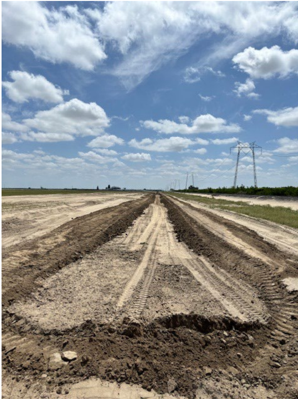
Sloping Sides of 4-ft Deep Keyway
