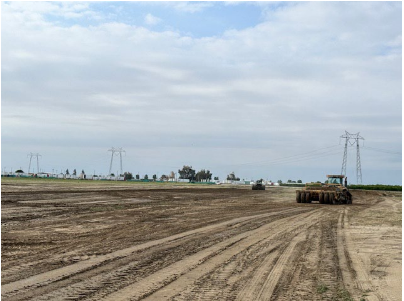
Backfill and Compaction of Keyway to Original Grade
