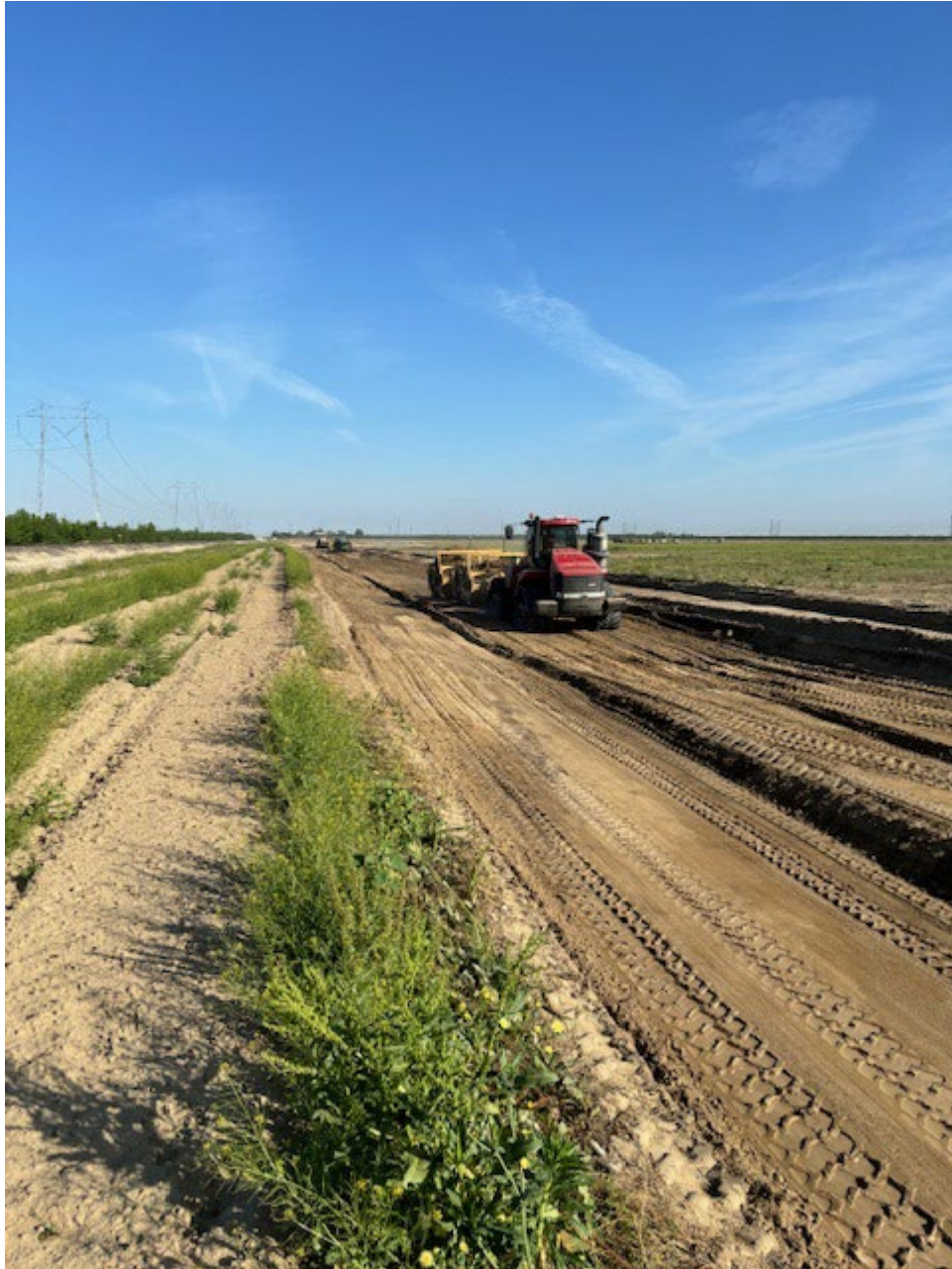
Excavation of Keyway along Westerly Levee of Basin 2
