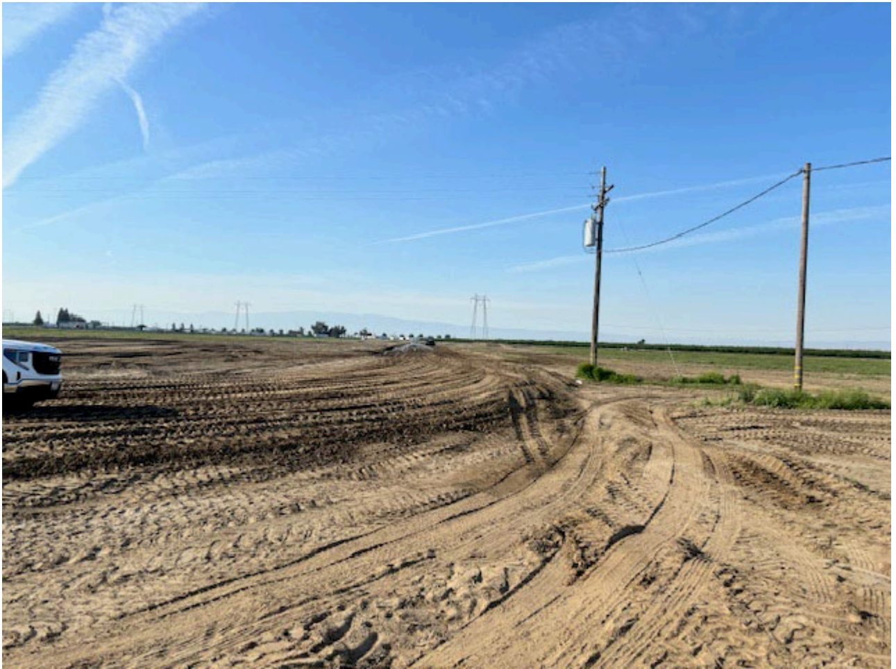
Backfill and Compaction of Keyway for Westerly Levee of Basin 1
