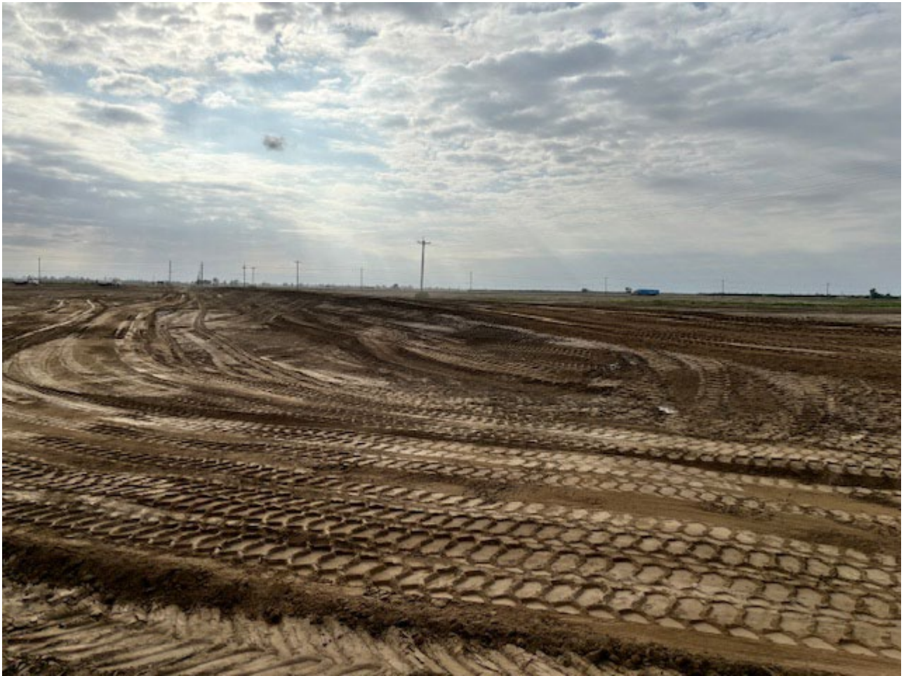
Levee Embankment Fill of Basin 1 – Basin 2 Northerly Levee Looking East
