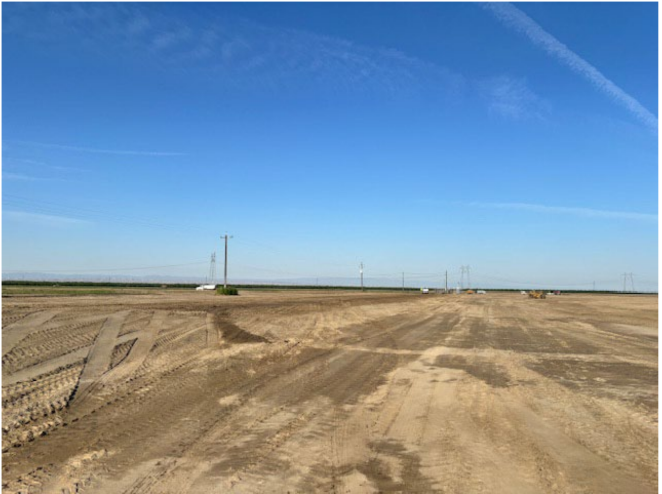
Backfill and Compaction of Levee Embankment for Northerly Levee of Basin 1
