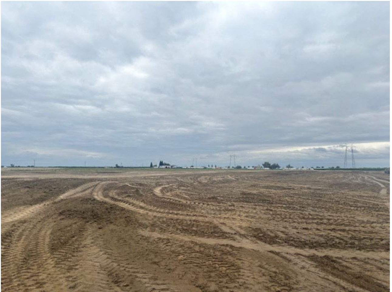
Levee Embankment Fill for Westerly Levee of Basin 1
