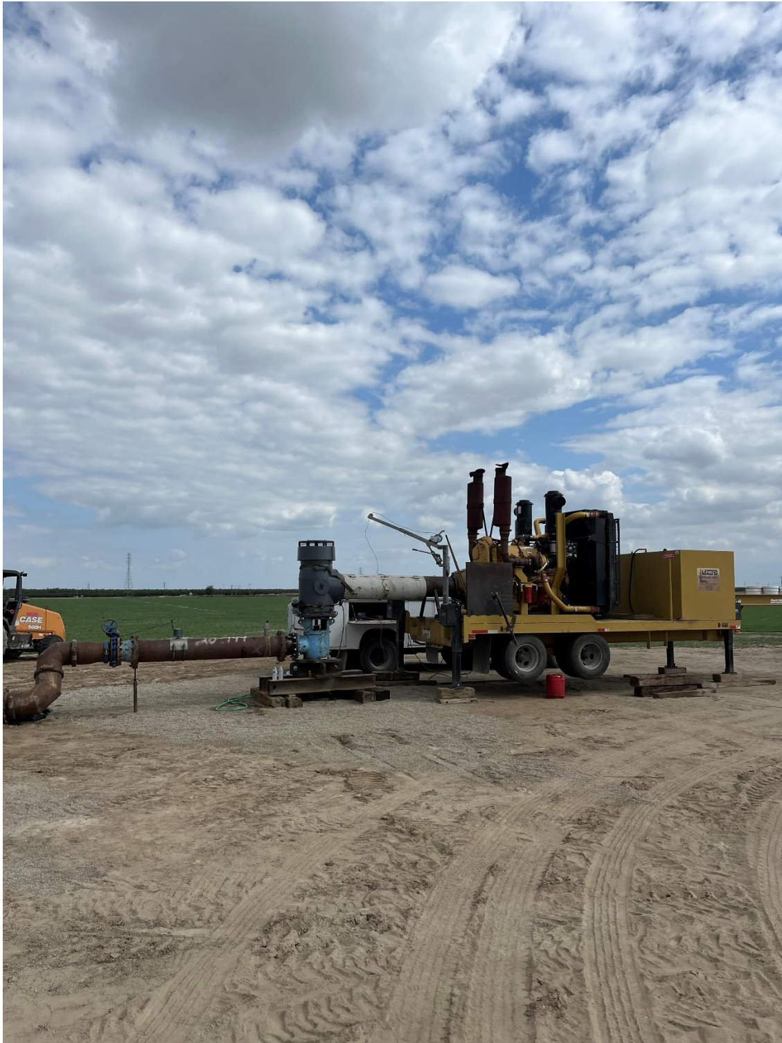
Figure 1: Diesel pump used for well development and pump testing
